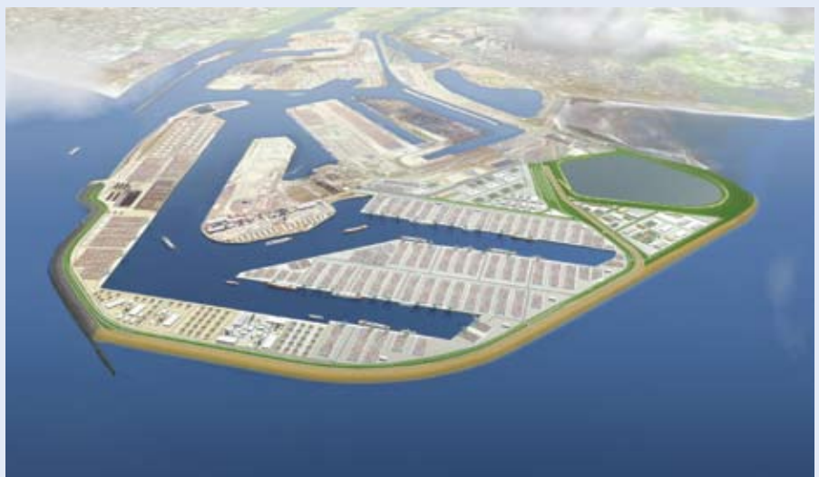
Construction of the Maasvlakte 2 has started
