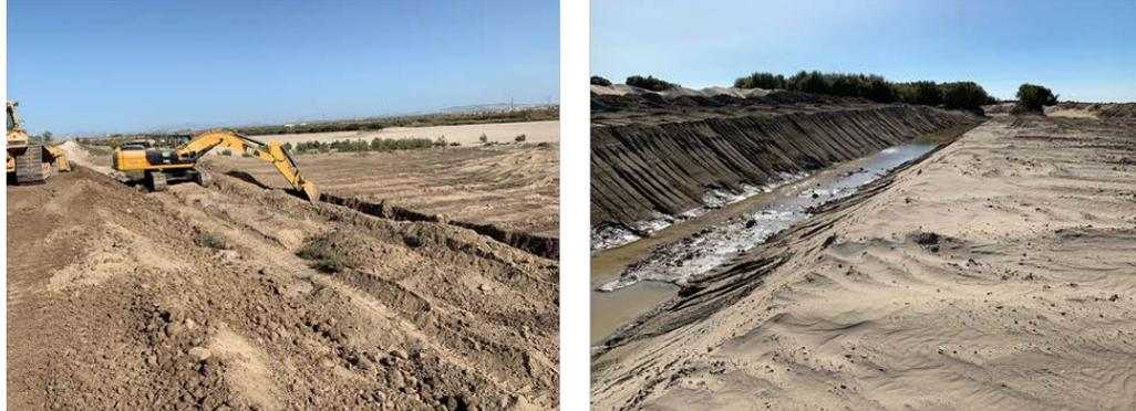
Figure 35. Channel construction in La Horcada Area
