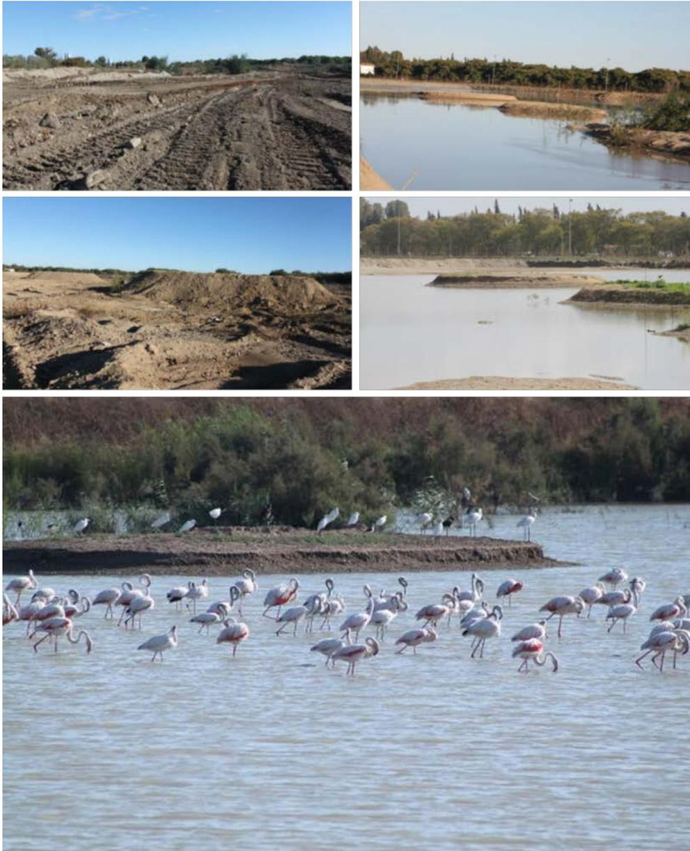
Figure 23. Confined disposal facility (CDF) of Butano at different stages of the annual cycle of dredging-disposal-extraction-adaptation. Source: Port Authority of Sevilla
