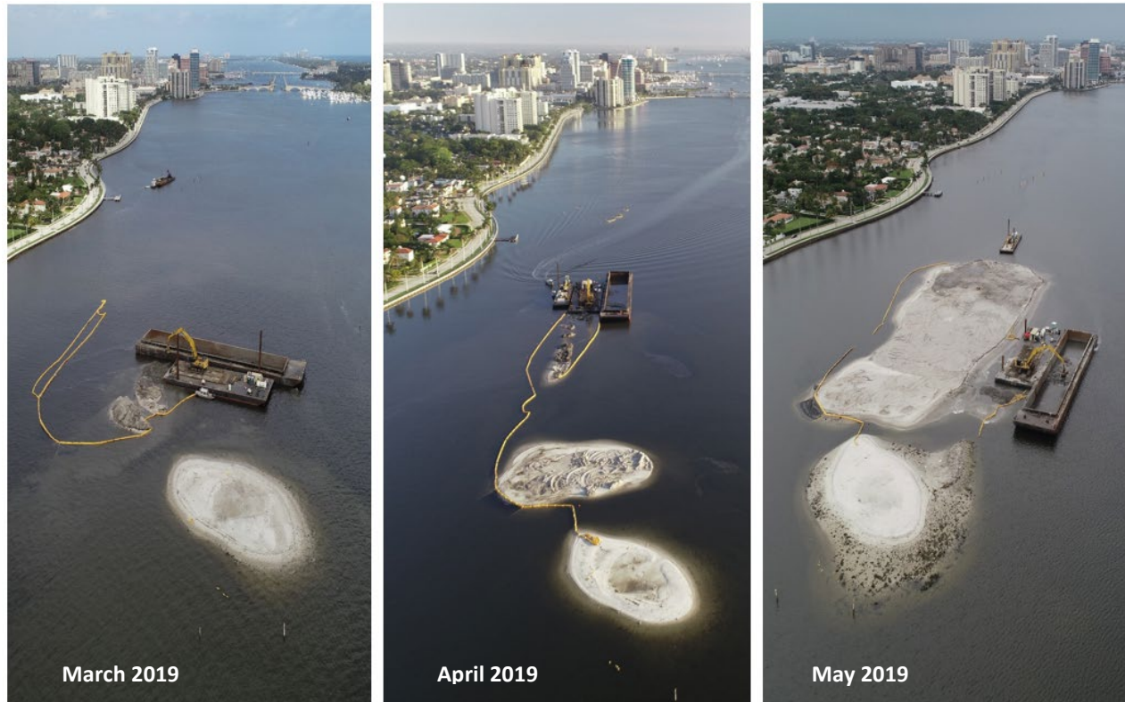
Figure 6. Tarpon Cove Restoration Area During Project Construction
