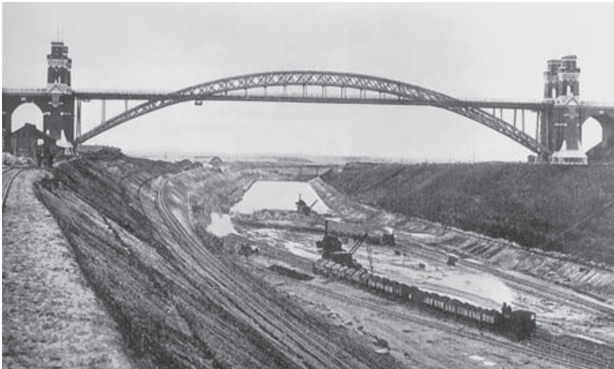
The Kaiser Wilhelm or Kiel Canal connects the North Sea and the Baltic Sea and shortens the voyage between the two seas by almost 500 km. Construction started in 1887. Large steam excavators and small steam trains were used to dig the canal. After eight years, on 21 June 1895, Emperor Wilhelm II was able to inaugurate the canal.
