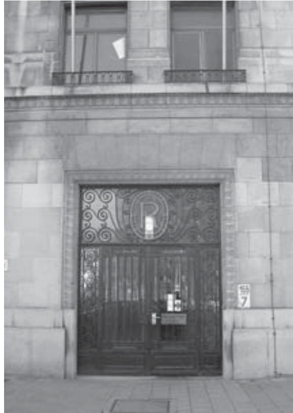
The entrance of the Jugendstil Residence Palace, 155 Rue de la Loi, was the postwar office of PIANC. In 1991, PIANC Headquarter moved with the Belgian Ministry to the World Trade Centre near Brussels North Station.
