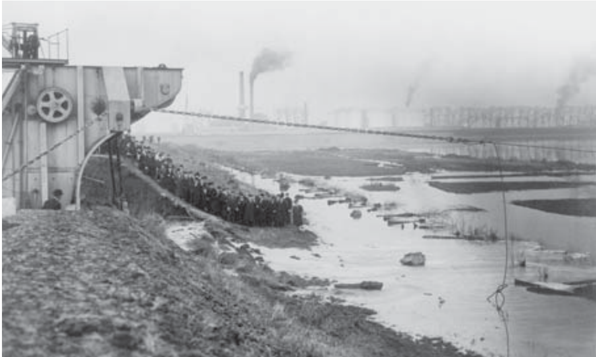
A special moment, watched by many spectators: a bucket dredger ploughs its way through a dike in order to construct a new harbour basin, in this case the Rotterdam Walhaven.
