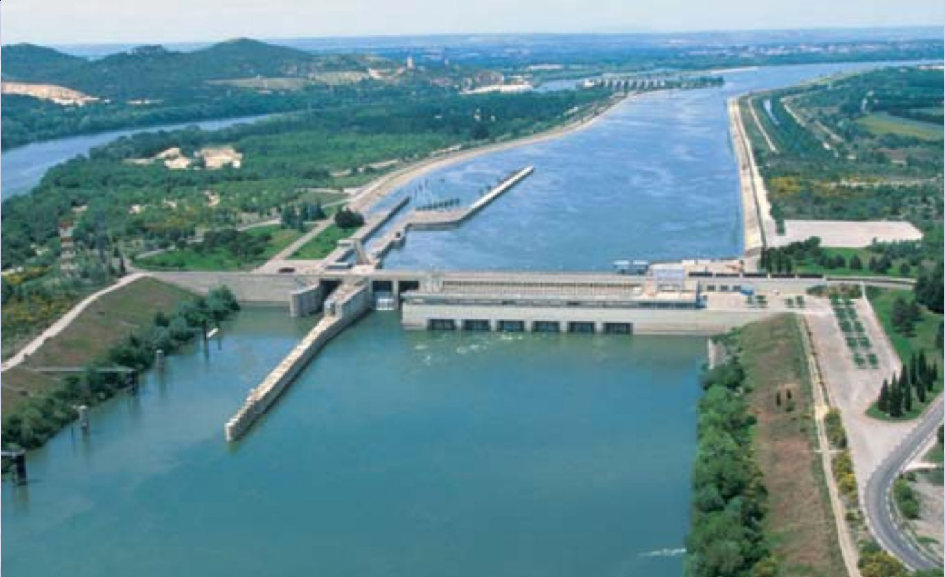
The River Rhône has been equipped with locks and dams to generate hydropower and water for irrigation and to improve navigation. The photo shows a lock and dam in an agricultural area near Vallabrègues. At the left is the lock for navigation.
