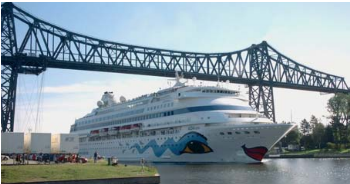
The bridges across the Kiel Canal once looked very high. Today, their height is hardly enough to allow passage of large passenger and container vessels.
