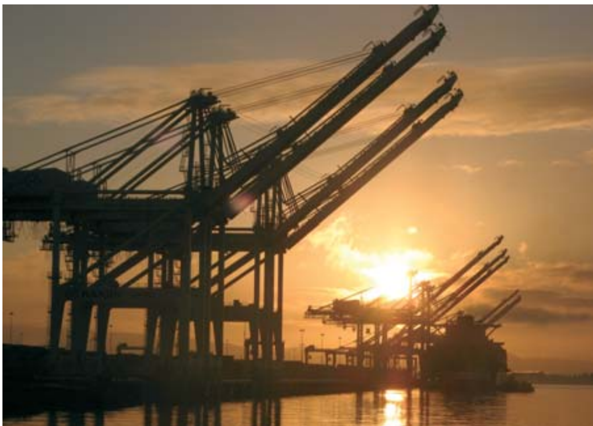
Today, containers and container cranes dominate the port skyline. The old-fashioned general cargo ship almost disappeared in favour of container ships.
