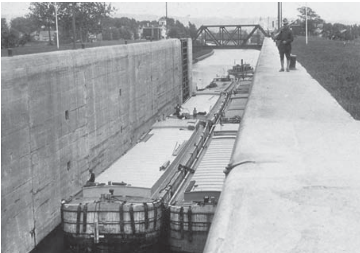
The Erie Canal connects Albany on the Hudson River to Lake Erie. The opening of the 580 km artificial waterway in 1825 caused a dramatic decrease in over-land transport costs. Originally barges were towed by mules. This photo of lock 3, taken in 1918, shows a steamboat. The canal's peak year was in 1885 with 33,000 ship movements. Today the canal is mainly used for recreational purposes.
