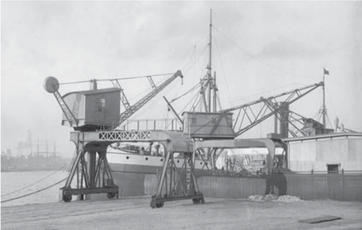
Shortly after 1890 electric cranes made their appearance. They had many advantages over the steam and hydraulic cranes of those days : less heavy machinery, flexible positioning along the quayside, efficient with regard to energy and much cheaper per hour to operate.
