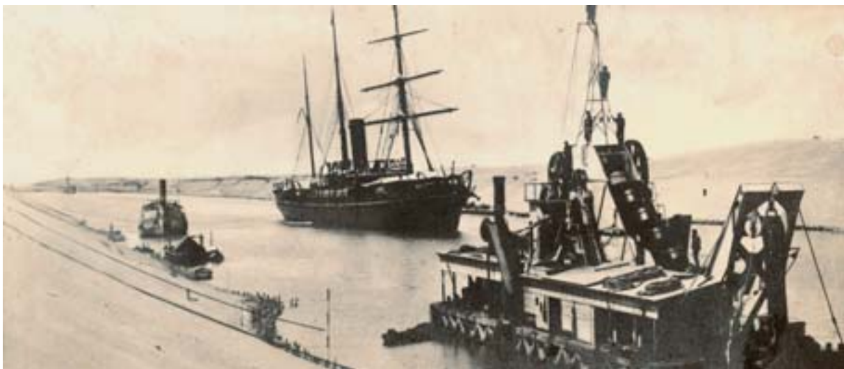
The Suez Canal, opened in 1869, was a major driving force for the development of steam navigation, because sailing was not allowed on the canal. The waterway was enlarged several times as ships grew bigger and bigger, but it needed continual maintenance dredging.
