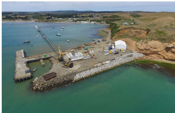
Figure 9 - Waitangi Wharf upgrade during construction in Jan 2017
