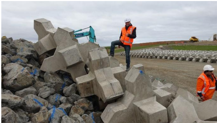
Figure 5 - Xbloc placed on a test slope
