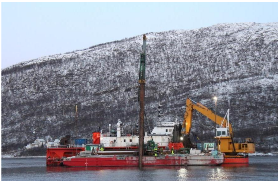
Picture 2. Positioning of pile - Kvalsundet (photo: NCA).
