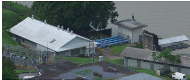
Figure 7: Paraiso Intake Station
