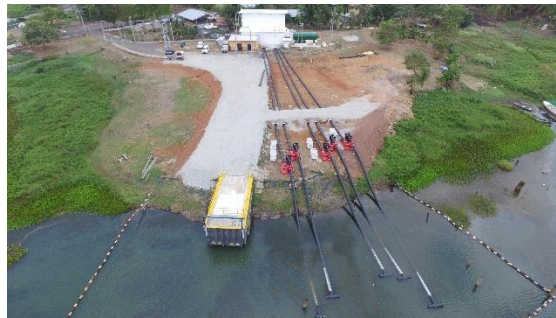
Figure 10: Mendoza Filtration Plant intake at Gatun Lake
