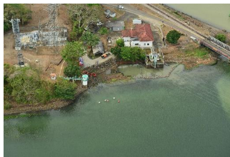
Figure 6: Gamboa Intake Station At Chagres River
