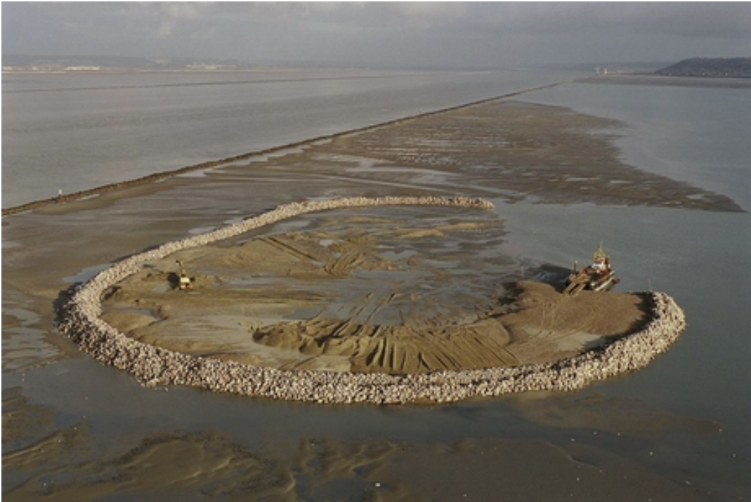
Figure 4. Bird Island constructed using dredged sediment.
