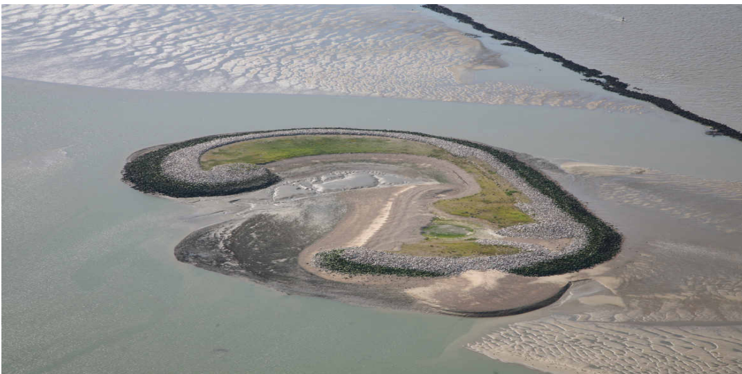
Figure 4. Bird Island constructed using dredged sediment.
