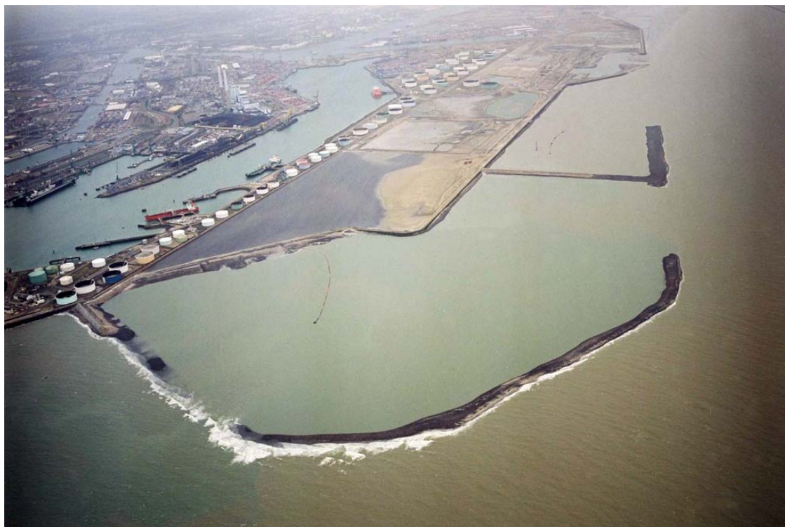
Figure 3. Breakwater sub-base made of gravel
