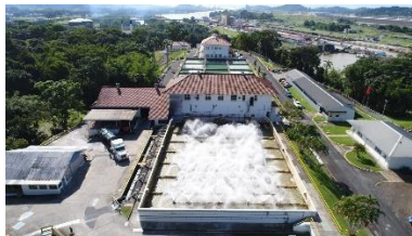
Figure 5: Miraflores Filtration Plant 2018.
