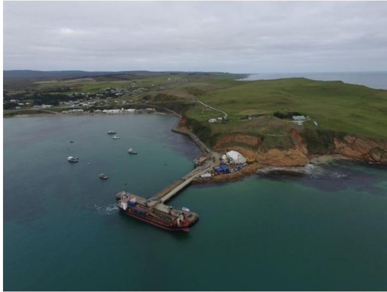
Figure 3 – The existing wharf at Waitangi showing the T-shaped wharf and small operational area.
