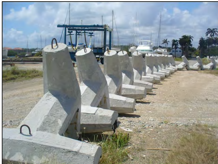
Figure 16: 8 tons dolosse used repair the Cristobal breakwater
