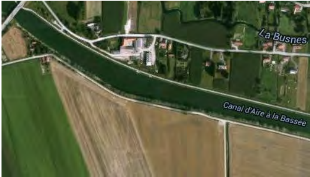
Figure 3: example of bend with the lack of an adequate width addition according standard design rules
