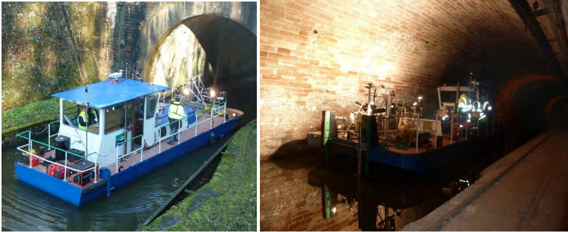
Figure 9: Our acquisition prototype mounted on a barge at the entrance of the tunnel (left) and inside the tunnel (right)
