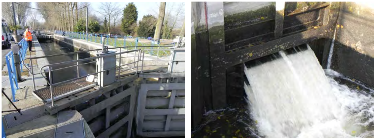
Figure 18: Lock of Leers-Nord: (a) General view; and (b) grid valve in the upstream gate
