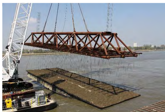
Figure 15: Immersion of the asphalt mattresses in front of the quay wall
