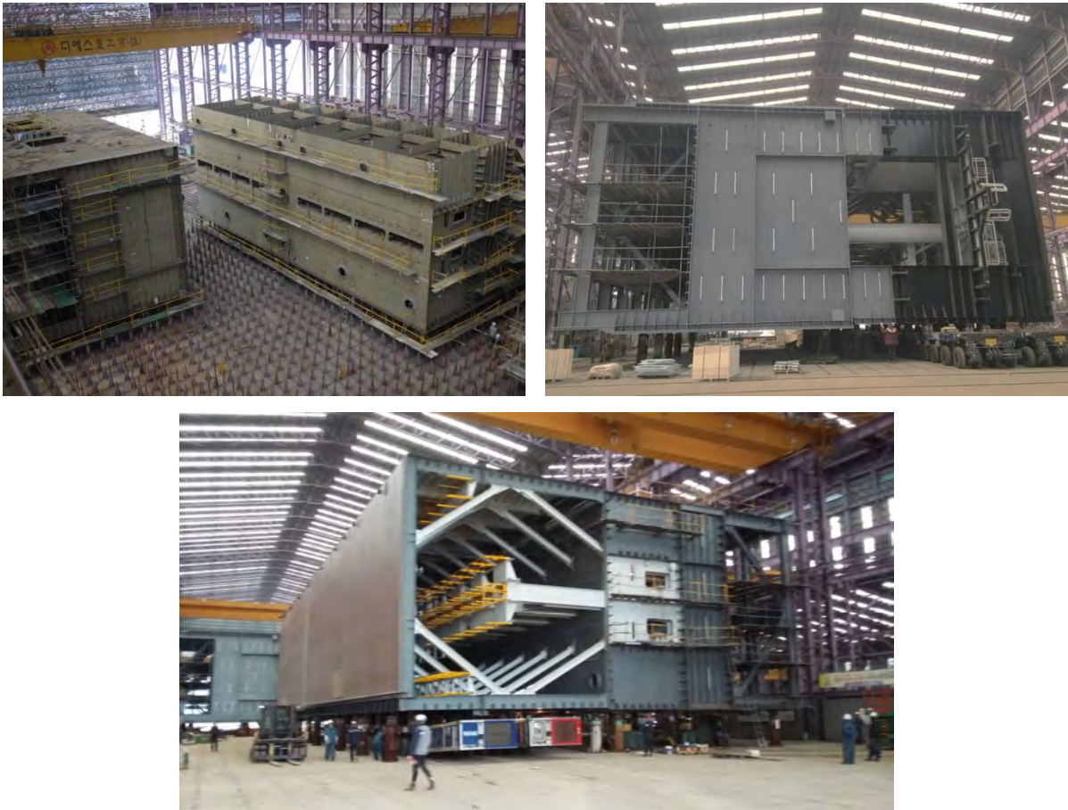
Figure 20: Steelwork fabrication of the lock gates in South Korea
