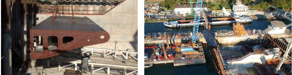
Figure 12 Le Coudray Weir: gate lifted to the cofferdam
