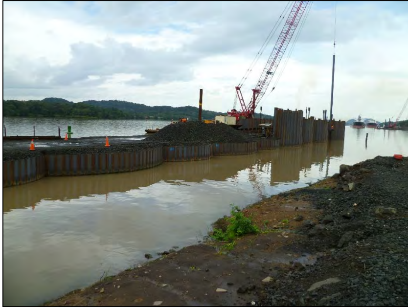
Figure 19: Filling operation of the cells
