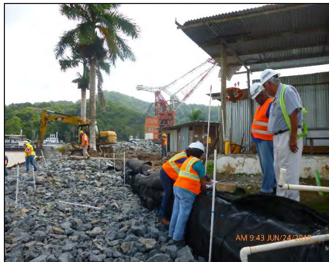
Figure 24: Anchor trench for the geocomposite
