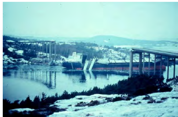
Figure 2: Tjörn Bridge Collapse, Almo Sound, Sweden (1980)
