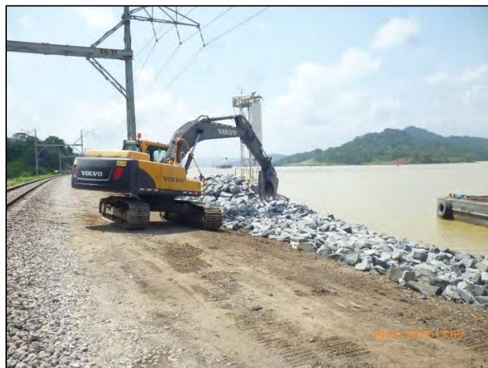
Figure 8: Placement of armor stone in site
