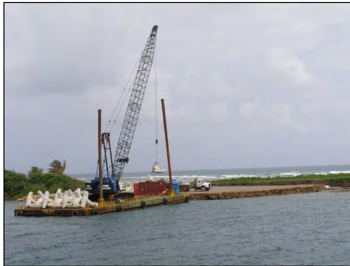
Figure 17: Placement of dolosse on the barge
