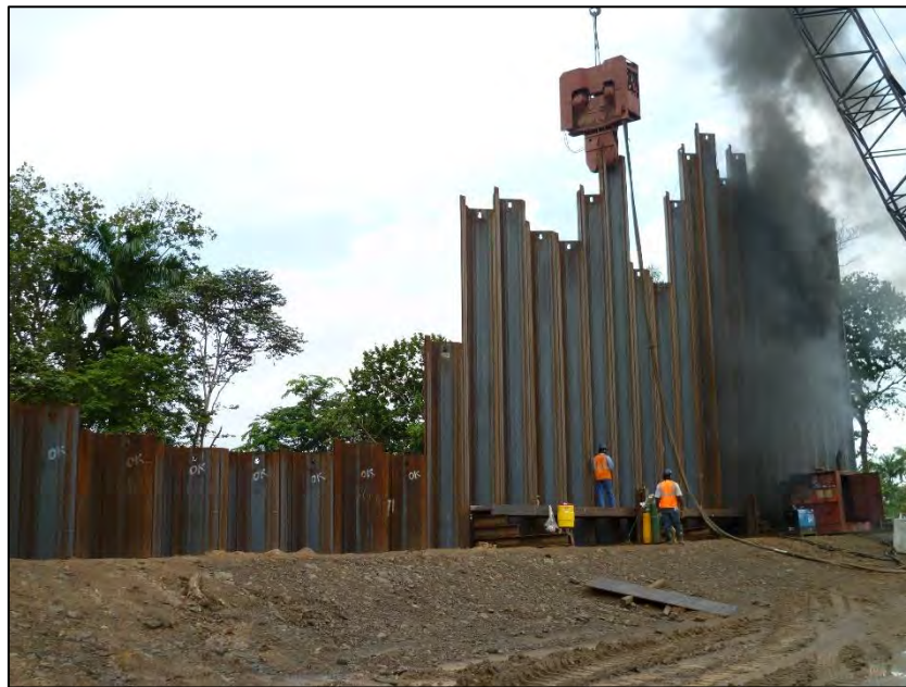
Figure 22: Driving sheet piles for the embankment cutoff wall
