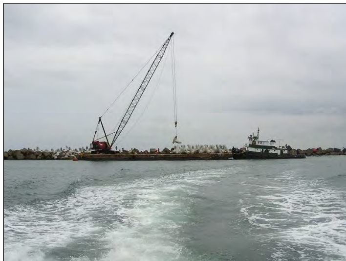
Figure 18: Installation of dolosse in the West breakwater
