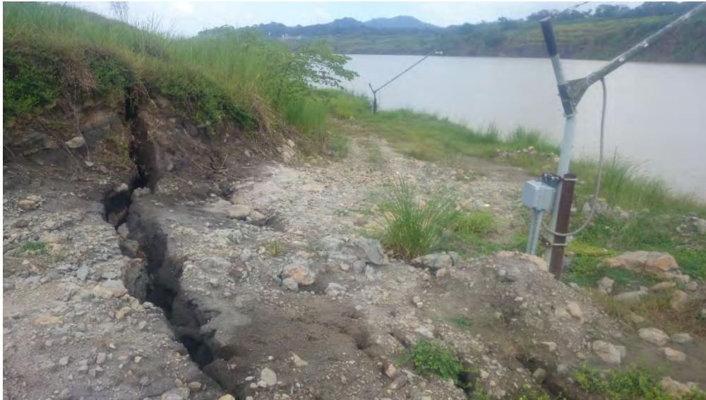
Figure 12: Tension Cracks at Old Lirio Slide Area
