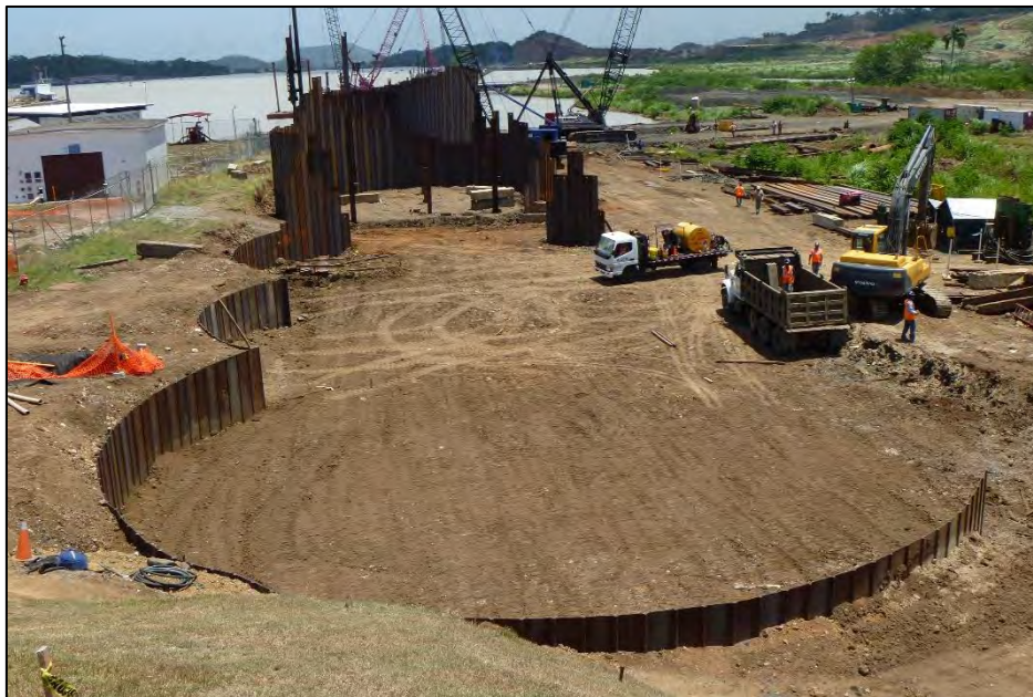
Figure 21: Landside cofferdam in the north end after cutting off sheet piles
