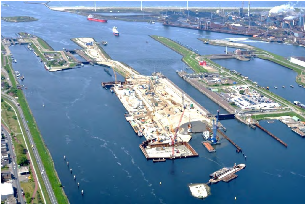
Figure 3: Construction site in the middle of existing lock complex (February 2018)
