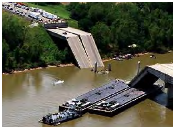
Figure 5: I-40 Bridge Collapse, Oklahoma, U.S. (2002)
