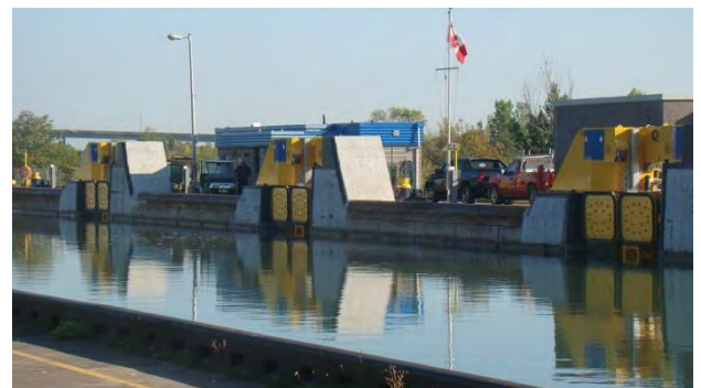
Figure 5: Mooring units centered in the lock wall, 25 m apart from each other
