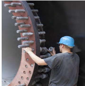
Figure 9 - Chatou gate : gate in the cofferdam - bolting - bound tubes
