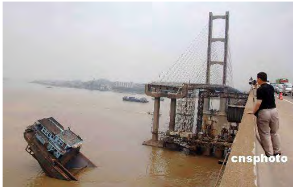
Figure 3: Jiujiang Bridge Collapse, Xijiang River, Foshan, China (2007)
