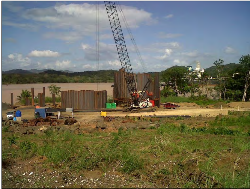
Figure 20: Landside cofferdam in the south end
