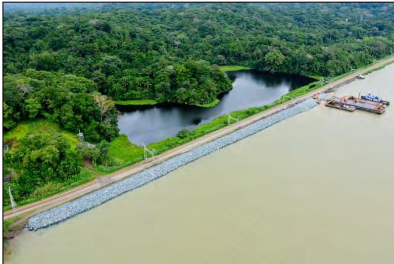
Figure 10: Plan view showing the project finished
