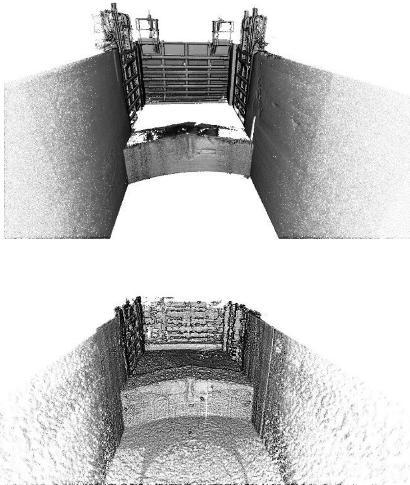
Figure 5: Laser (top) and sonar (bottom) models of the upstream lock gate
