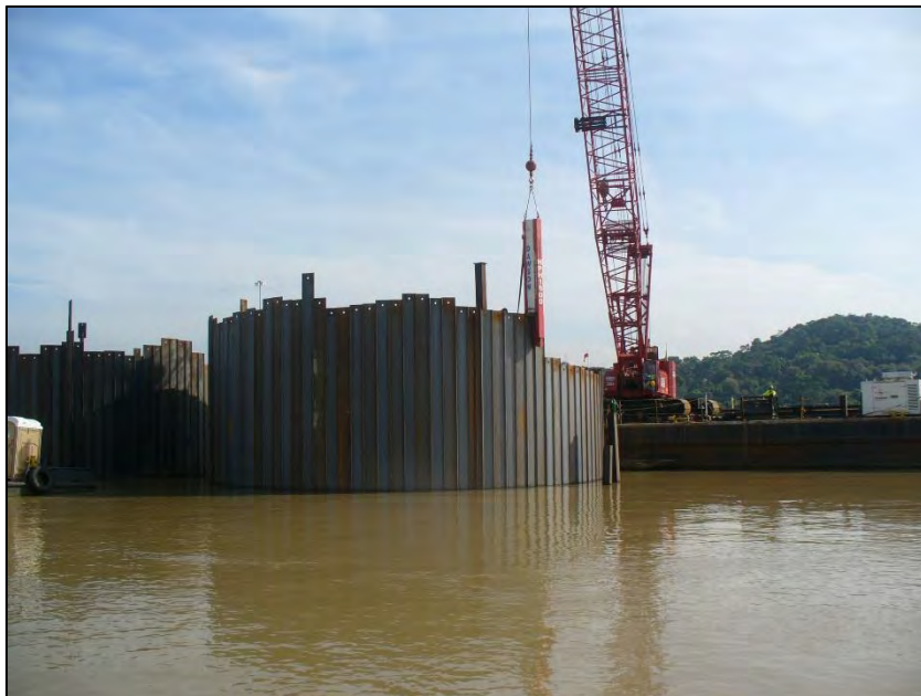
Figure 18: Driving piles in a cell by vibration
