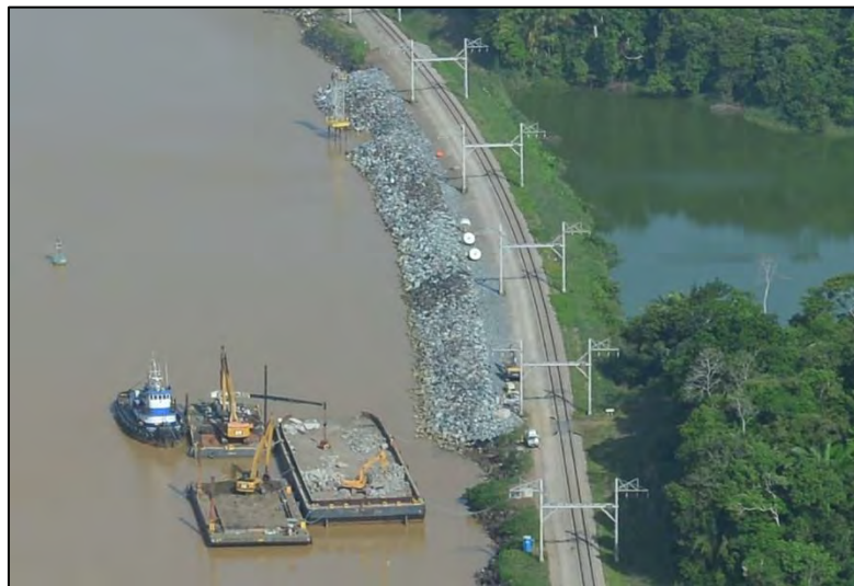
Figure 7: Transportation of the armor stone
