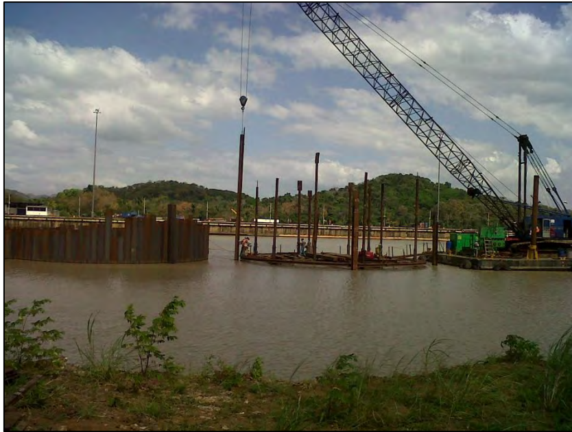
Figure 17: Template in position
