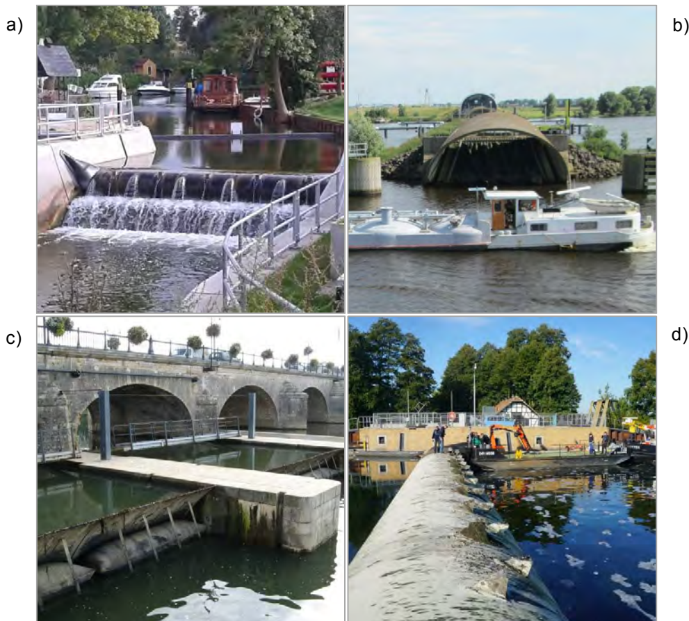
Figure 2: Applications of inflatable gates at waterways
