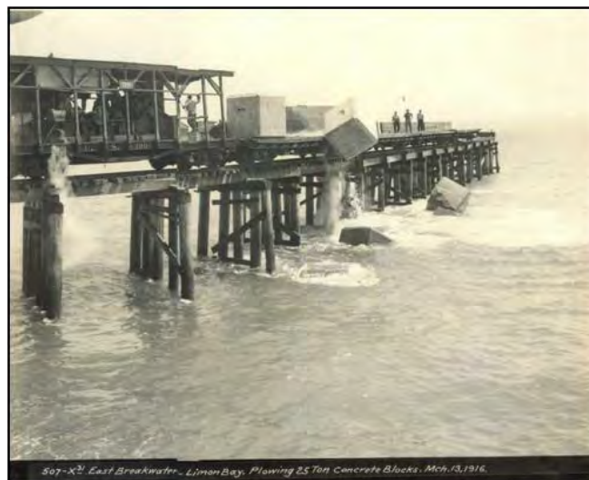
Figure 15: Concrete blocks dumped for the shell of the East breakwater
