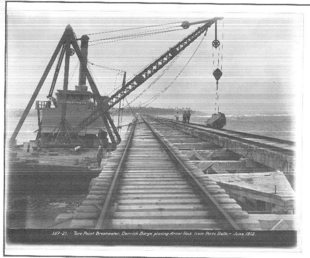
Figure 14: Rock blocks for the shell placed by a crane
