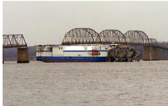
Figure 4: Eggner's Ferry Bridge Collapse, Kentucky, U.S. (2012)
