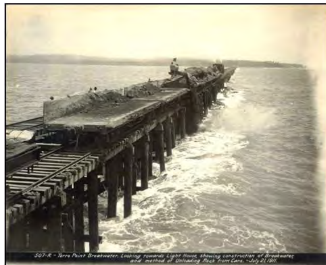
Figure 13: Material for the core being dumped from the train
