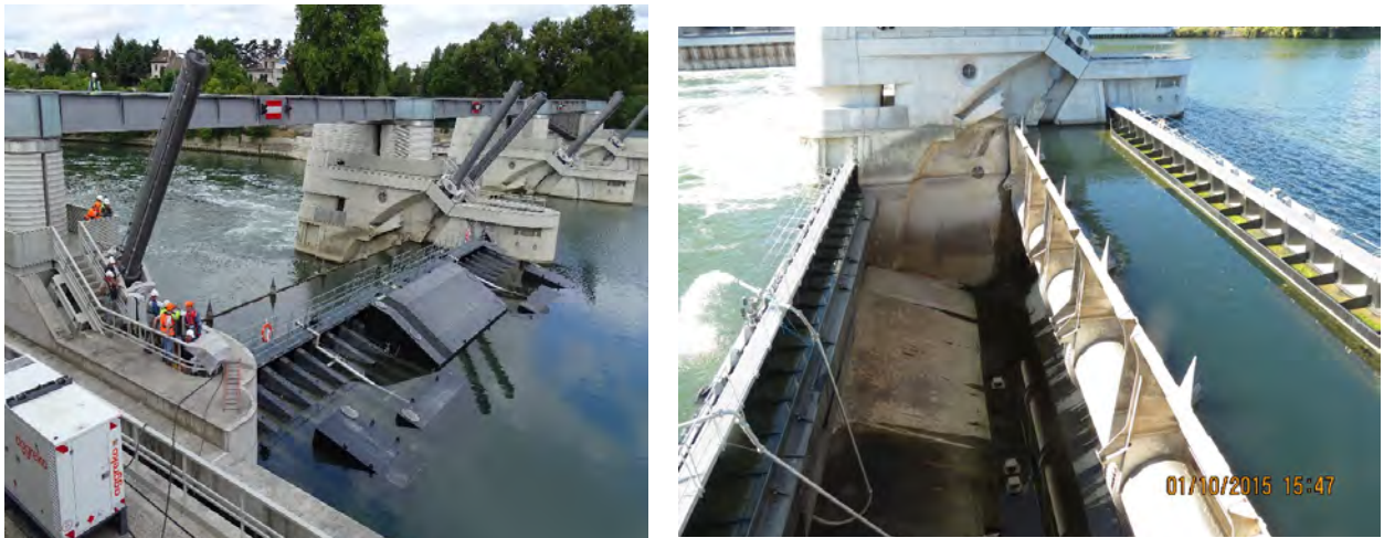
figure 21 - Chatou Bulkhead arriving by buoyancy and in final position (first use)
