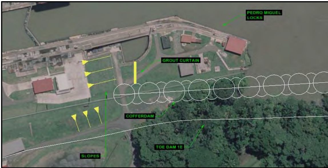
Figure 3: North tie-in of cofferdam (at Pedro Miguel Locks)
