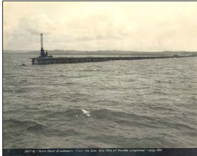
Figure 12: Pile driving and trestle assembling
