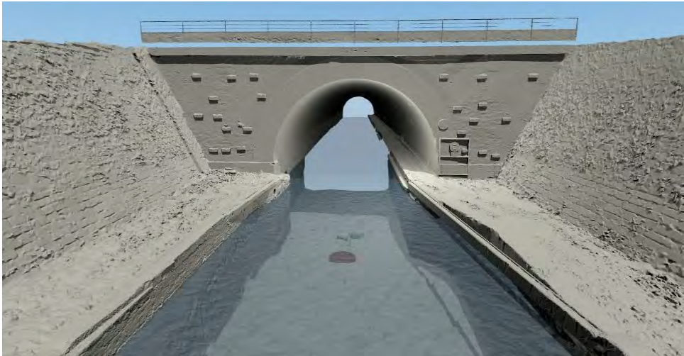
Figure 17: Reference model of the west entrance of the canal tunnel. The dark disk in the middle of the canal indicates the location of the MSS station
