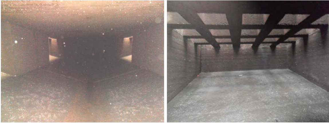
Figure 2: Lock of Havré. Views from inside the central diffusion culvert.
