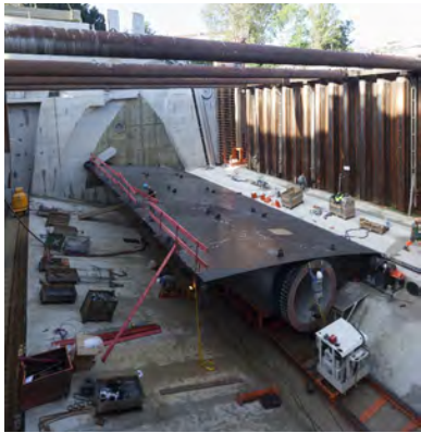
Figure 9 - Chatou gate : gate in the cofferdam - bolting - bound tubes
