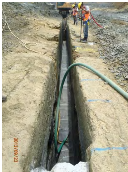
Figure 8. Cleaning of concrete cutoff wall trench
