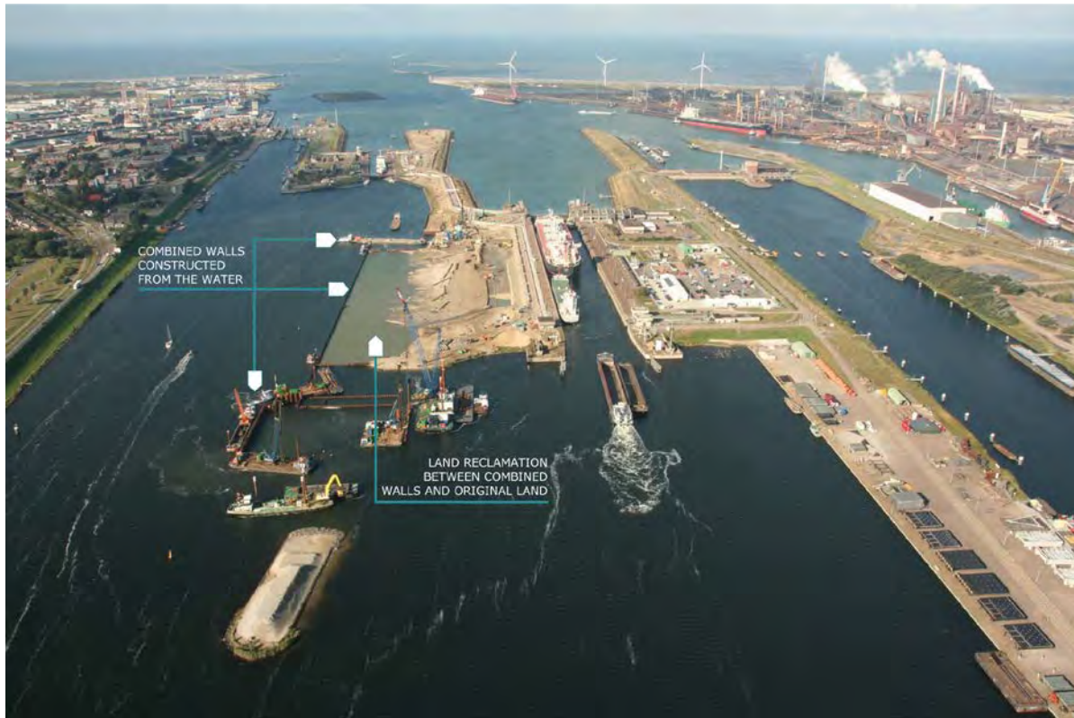
Figure 15. Construction of new lock in IJmuiden, Combined wet-dry construction method.
