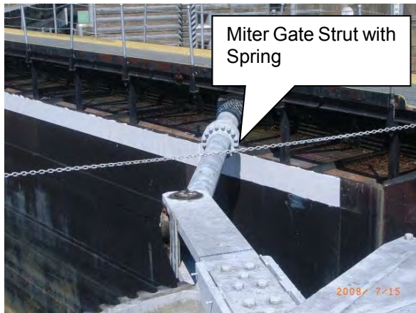
Fig. 13: Miter Gate Strut Spring
