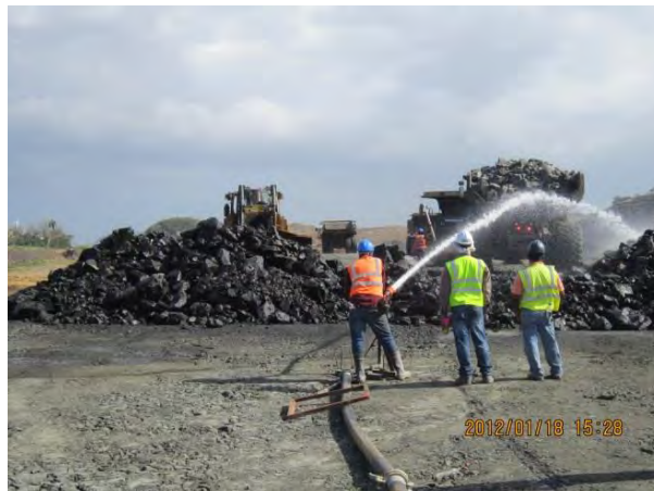
Figure 14. End-dumping, spreading, and watering of shoulder rockfill
