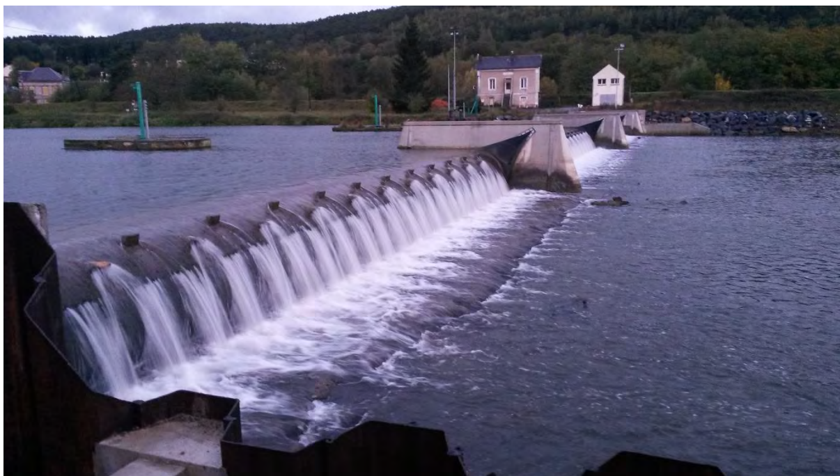
Lock 57 Ham. Inflatable rubber weir in operation. The original stake weir has been removed. It was further upstream of the new weir and its position is marked by the piers still visible.
