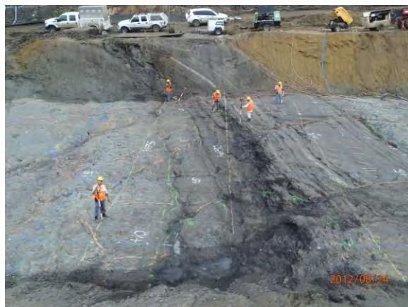
Figure 7. Geologic mapping of the dam core foundation
