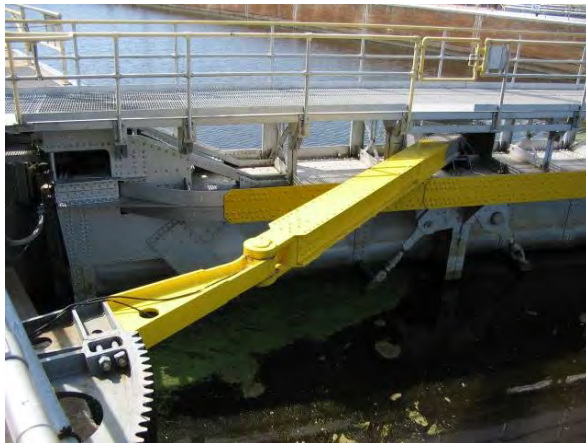
Fig. 14: Miter Gate Strut Assembly
