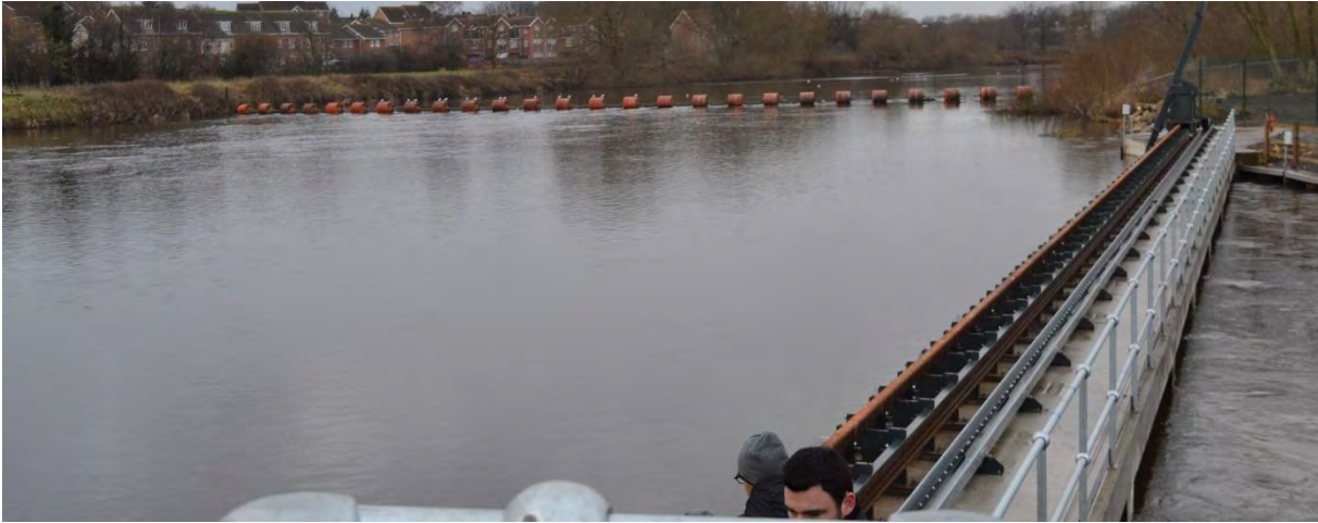
Knottingley Hydro Plant, Aire & Calder Navigation. Showing the large intakes necessary and the screen wiper at the upstream end.
