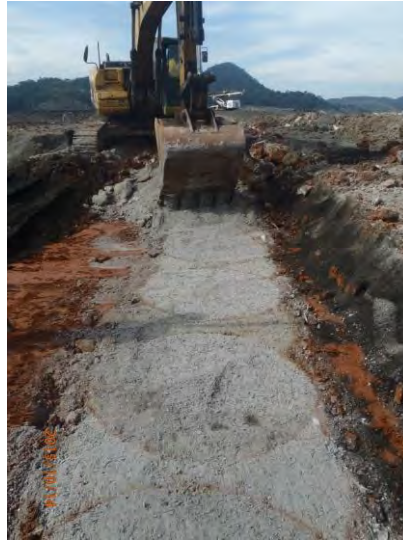
Figure 18. Trimming the top of the cutoff secant-pile wall
