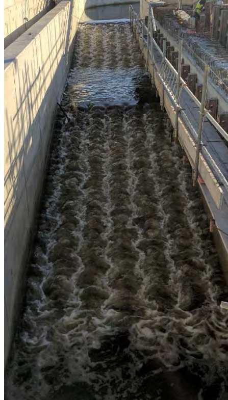
Larinier super-active baffle type fish pass under construction and in operation on the Aire & Calder Navigation in England – Pictures from Yorkshire Hydropower Ltd.
