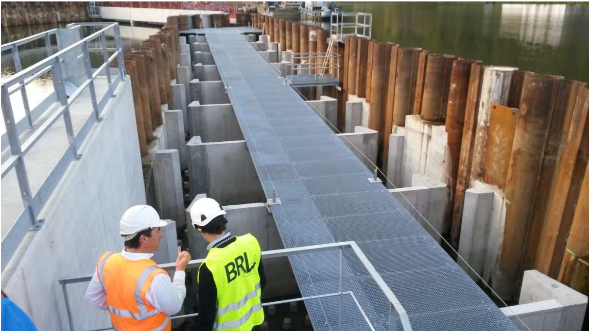
Lock 51 Saint Joseph. Fish pass of the double vertical slot type with bed substrate
