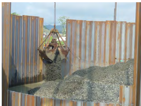
Figure 4. Backfilling of cellular sheet-pile segment of cofferdam
