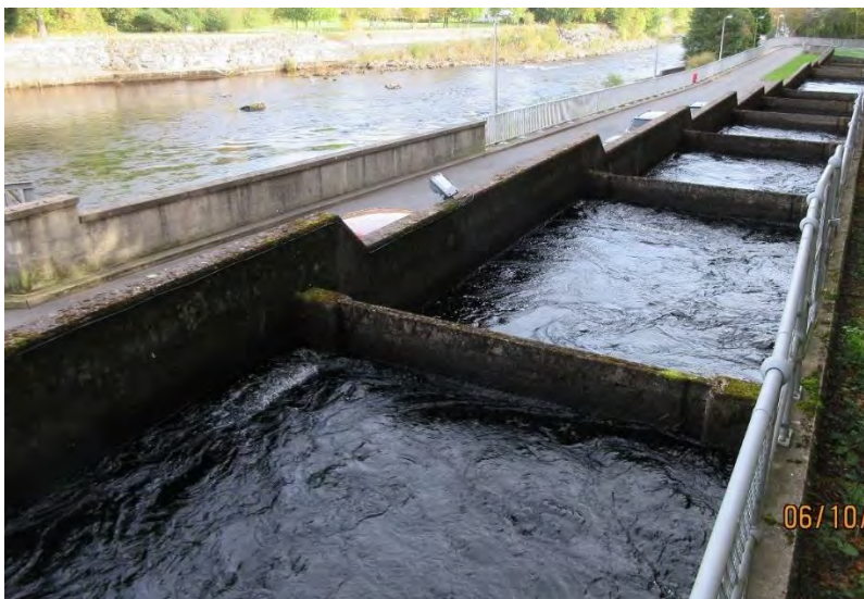
Pool fish pass in Scotland with submerged orifice
