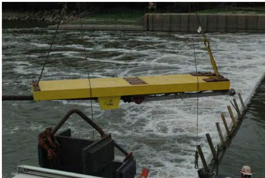
Figure 7: Installation of FRP Wicket Gate with UHMWPE
