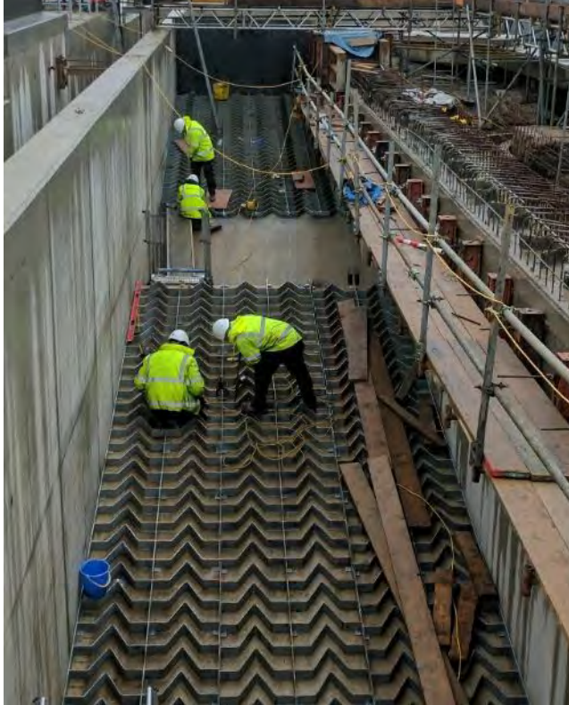
Larinier super-active baffle type fish pass under construction and in operation on the Aire & Calder Navigation in England – Pictures from Yorkshire Hydropower Ltd.
