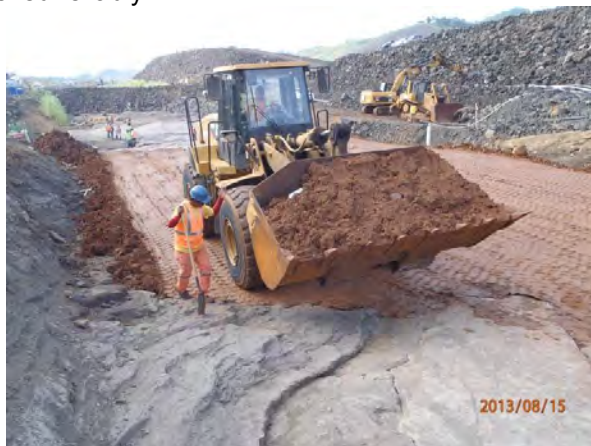
Figure 11. Compaction of core Zone 1A with front-end loader
