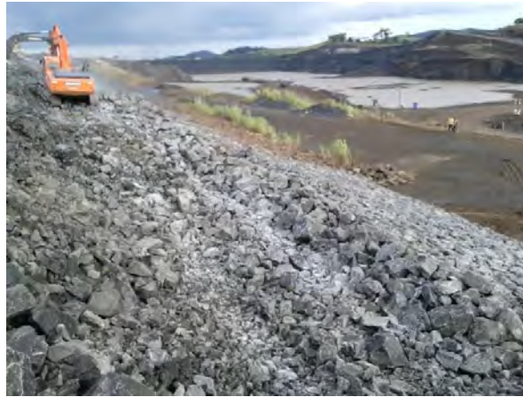
Figure 15. Riprap placement on trimmed face of rockfill
