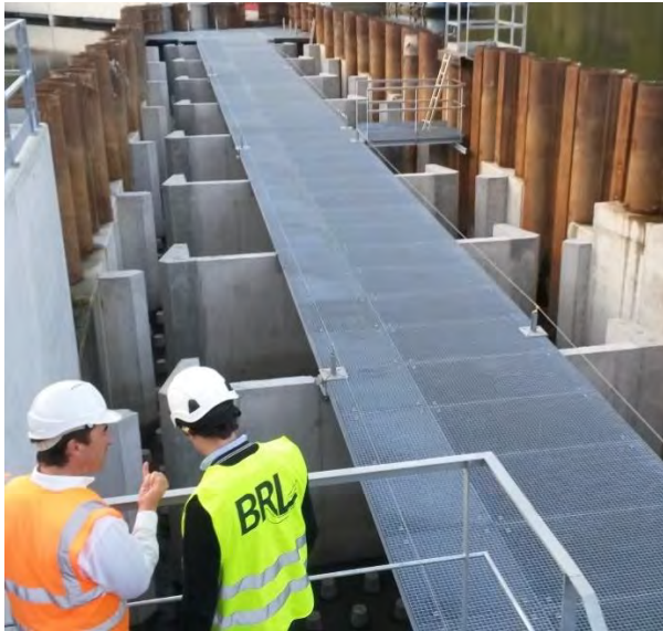
Pool fish pass in France with two vertical slots in each pool. The bed of the fish pass has additional moulded protrusions to assist the passage of benthic fish.
