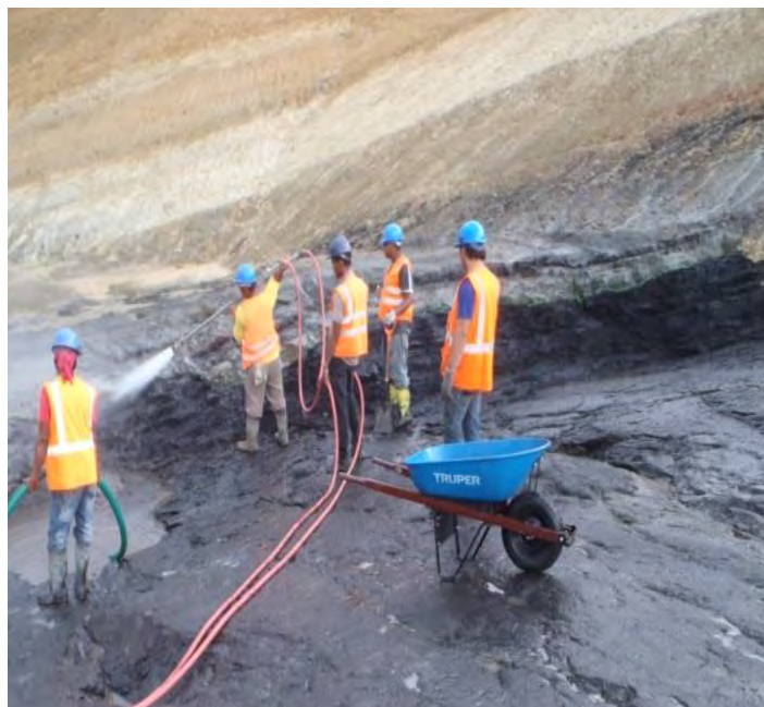
Figure 9. Cleaning of lignite bed for placement of backfill concrete
