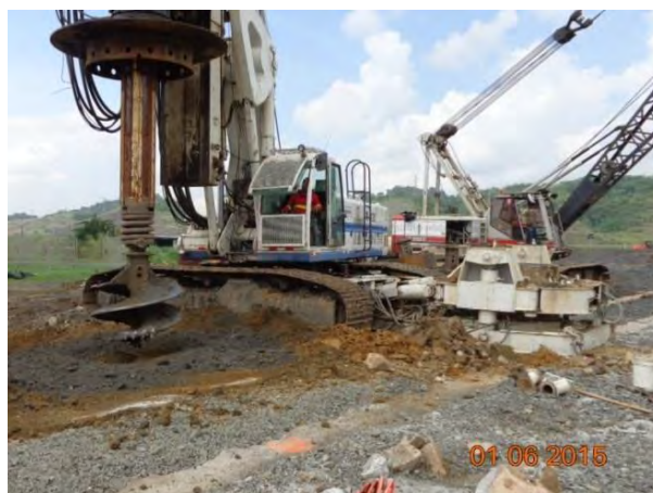
Figure 16. Excavation of secant piles
