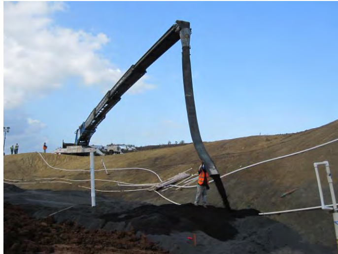
Figure 13. Placing filter material with telescoping belt and tremmie hose
