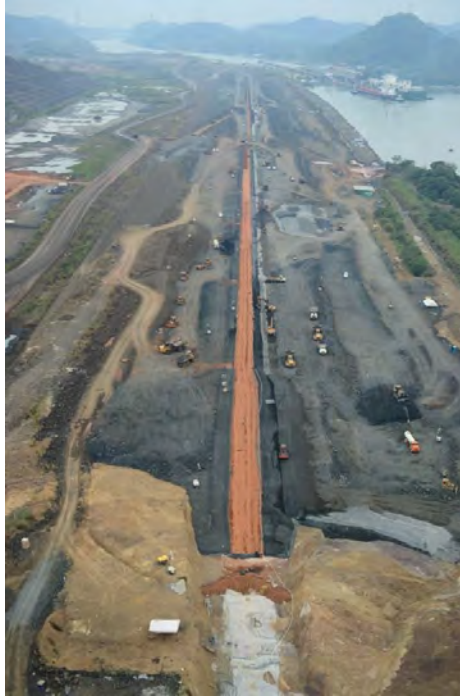
Figure 10. Dam embankment construction, looking north from Fabiana Hill
