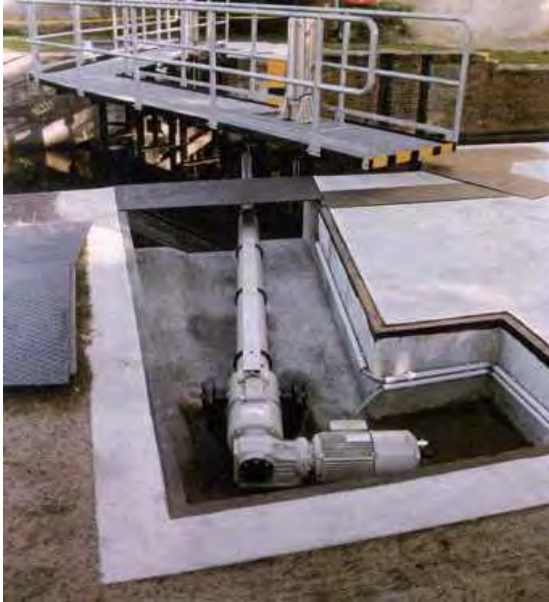
Fig. 7: Mechanical Linear Drive at a Miter Gate
