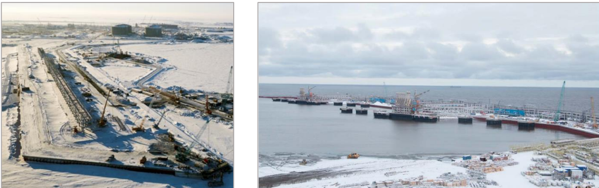
Figure 11: Construction of the South-West Breakwater and Ice Barrier & Main Export Jetties 1 & 2
