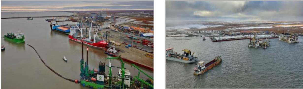
Figure 8: Dredging works in access channel near MOF
