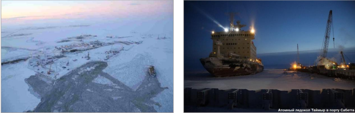
Figure 12: Ice management by ice-breaker during MOF construction
