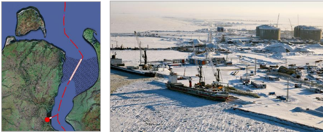
Figure 10: North Channel (left) and Construction of Marine Offloading Facilities
