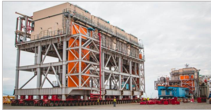
Figure 20: Module unloaded at Sabetta on a SPMT (Self-Propelled Modular Transporter)
