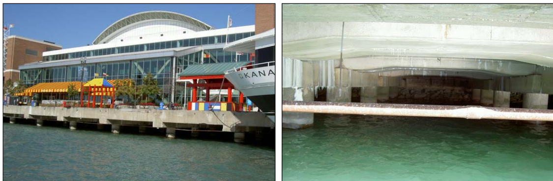
Figure 4. Existing deck-on-pile structure along the south side of Navy Pier.
