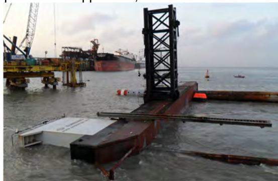
Figure 4: Pier III, Brazil
