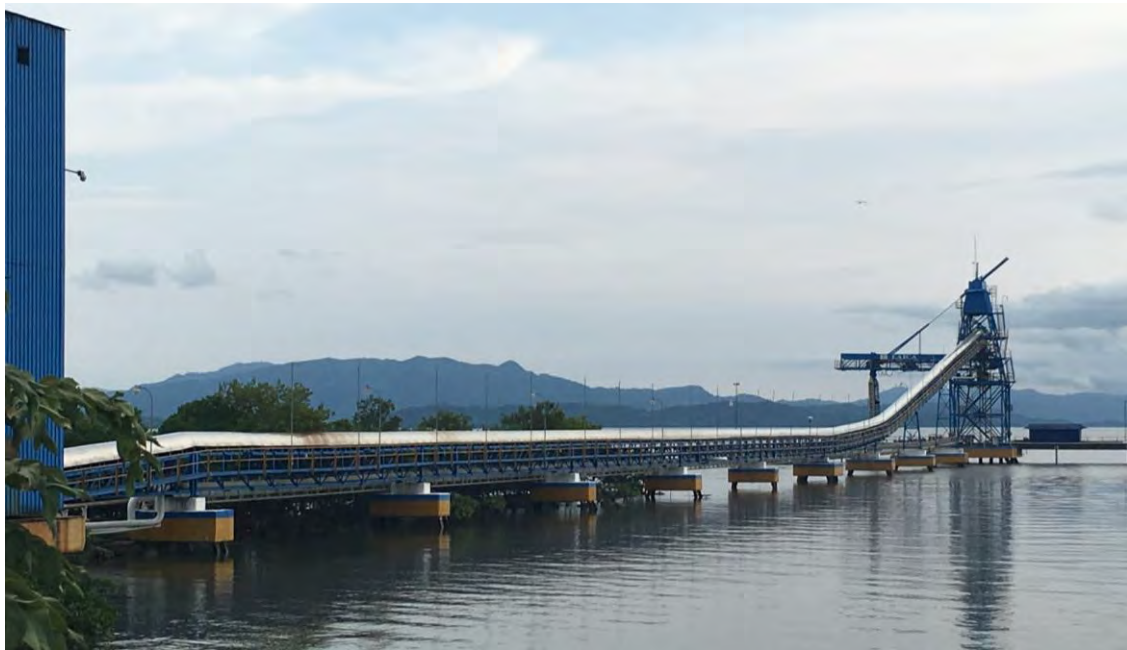
Fig. 17 Punta Morales Pier (Above) Layout of the pier including Charging Platform, Berthing Dolphins and Conveyor supports (Below) General View of Trestle Supports from land.
