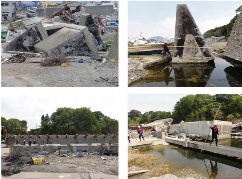
Figure 2: Images of tsunami-affected seawalls confirmed in the red-colored box area in Figure 1(b). (From the website of National Research Institute of Fisheries Engineering, Japan)
