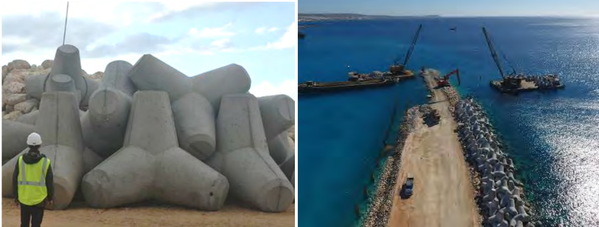
Figure 12. Test Cross Section in Land and Tetrapod Placement in the water.
