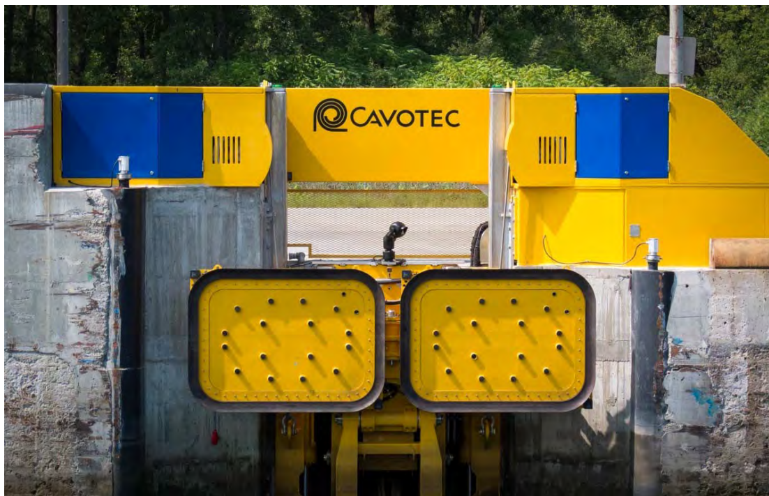
Cavotec MoorMaster™ MM400L 22 system installed in the St Lawrence Seaway, Canada
