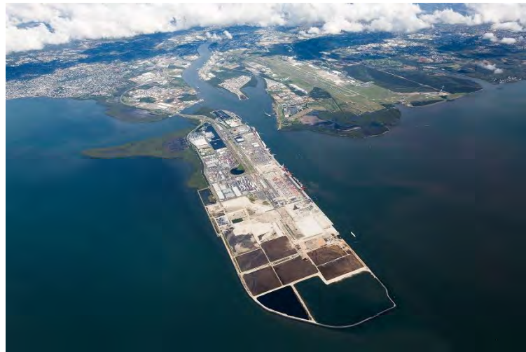
Figure 5 : The Port of Brisbane (PoB) is one of Australia's fastest growing container ports and Queensland's largest general cargo port. Port of Brisbane Pty Ltd (PBPL) is responsible for the maintenance and development of the port facilities as well as maintaining navigable access to the port for commercial shipping
