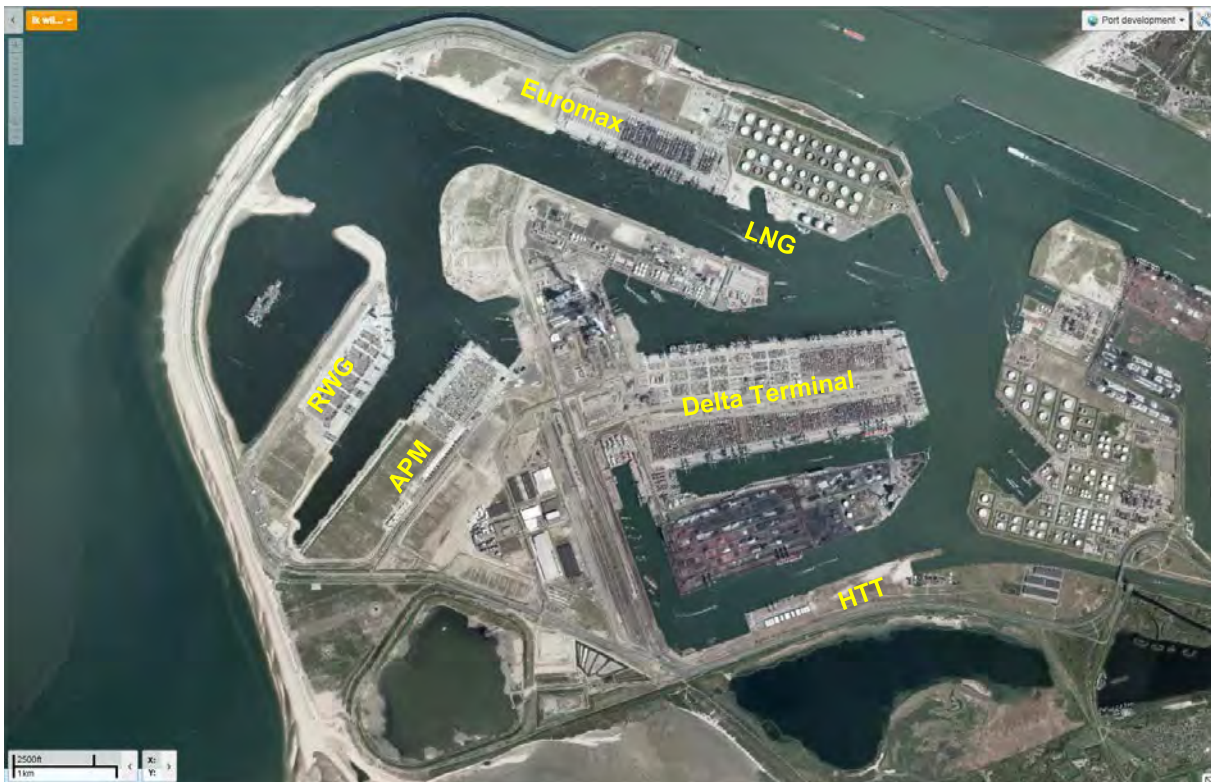
Figure 1: Overview Maasvlakte 1 and 2 with container terminals (photo PoR GIS database)
