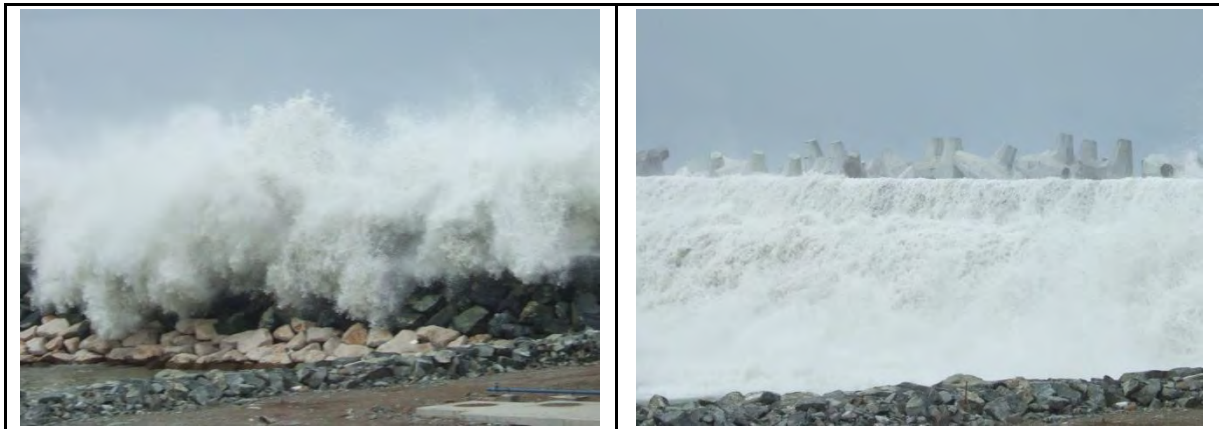
Figure 5 Heavy wave attack and overtopping on the south breakwater during TC Gonu
