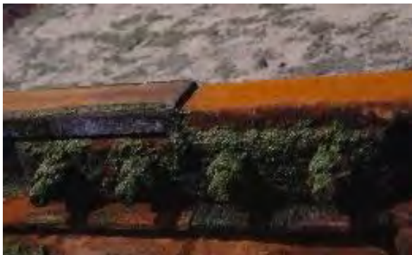
Fig: 27 Differential Aeration Cell Corrosion
