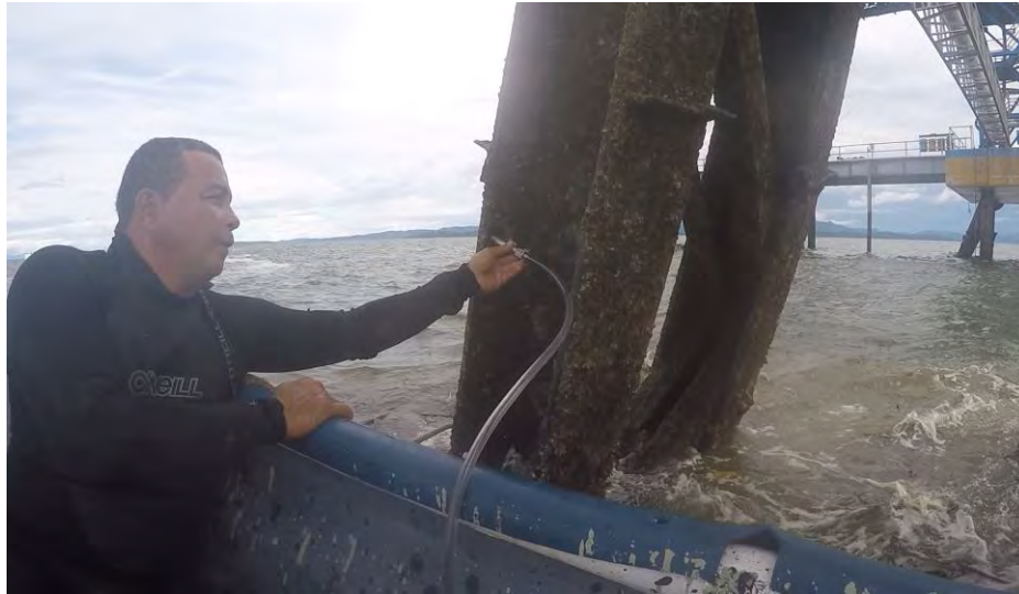
Fig. 19 Thickness measurement in one pile of the first support from the pier
