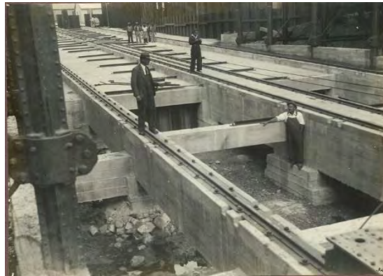
Fig 20: 1200 ton Slipway Construction in the Dry, Port Elizabeth 1945 – Military Specs!
