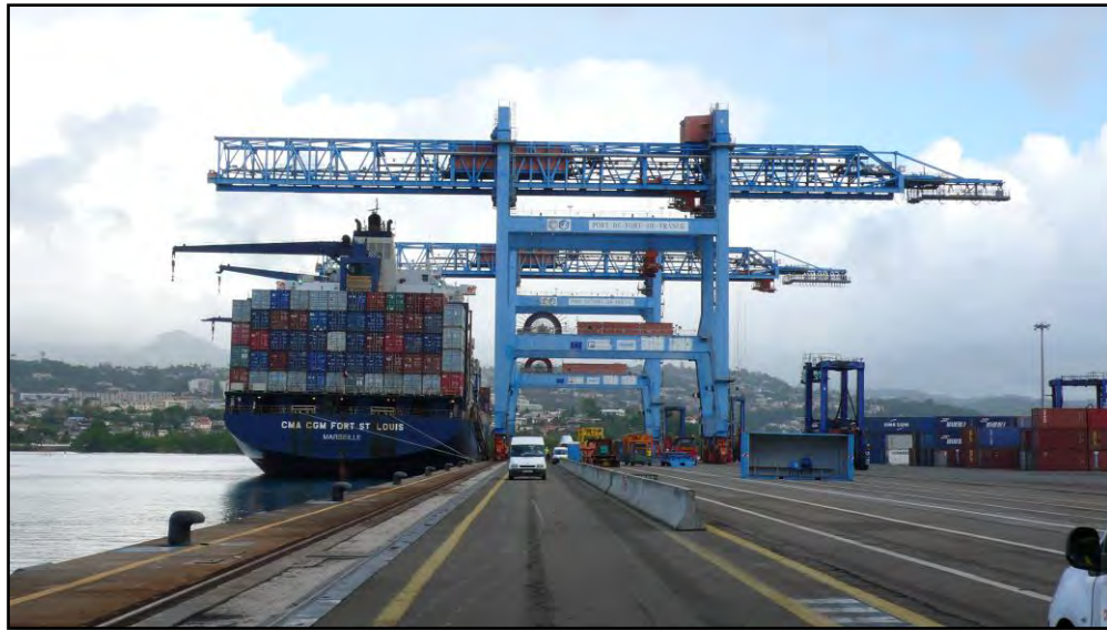
Figure 3: Pointe-des-Grives terminal gantry cranes in service (photo: Artelia)
