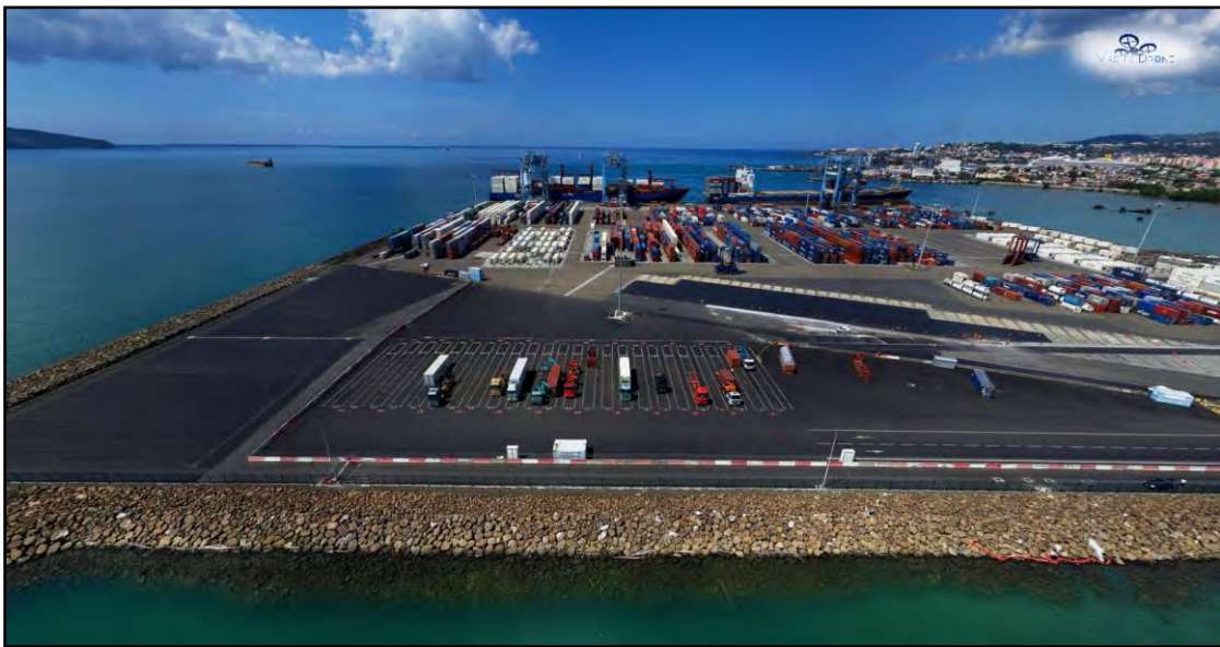
Figure 13: Aerial view of final reclamation area pavement (photo: Mad'In Drone (2017))
