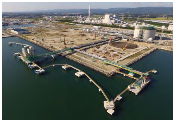
Figure 1: Aerial view of the receiving pier
