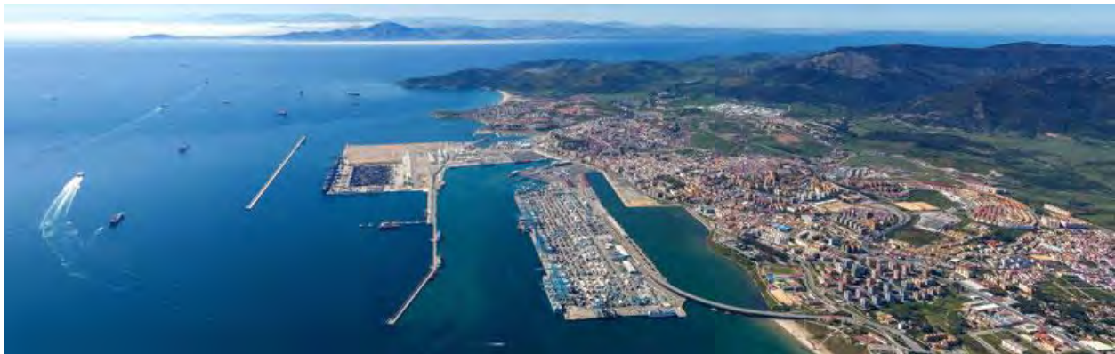
Figure 6. General view of Algeciras port.
