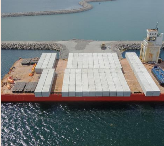
U1 protection beams
