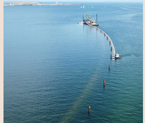
Pieline laying in western perimeter
