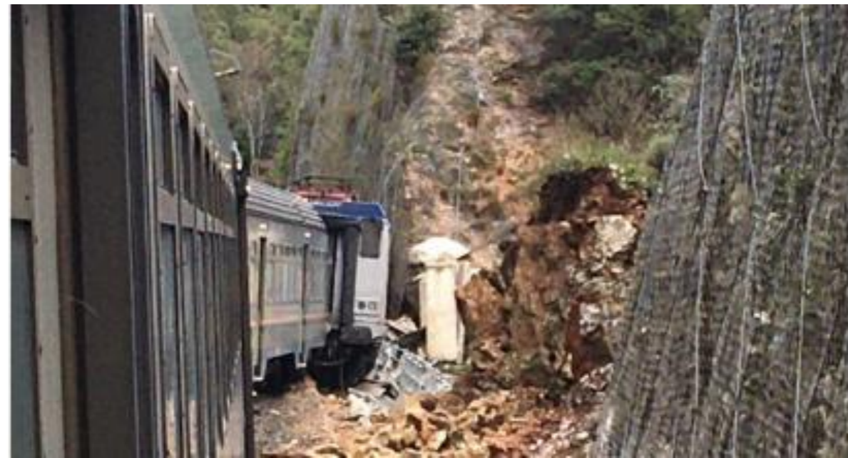
Landslide in 2021, Italy
