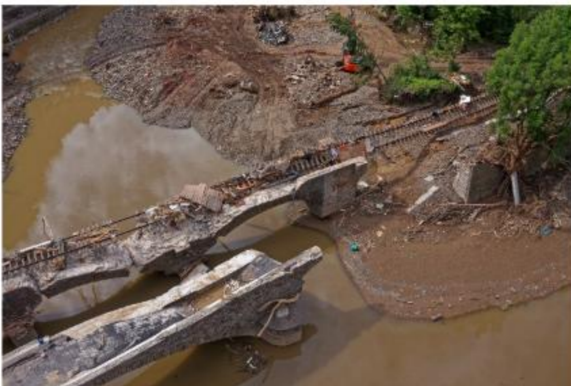
Bridge collapse in 2021, Germany
