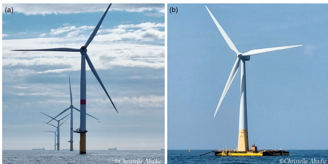
Figure 1: Examples of (a) bottom-fixed offshore wind turbines supported on a monopile (St Nazaire Wind Farm, September 2024), (b) the Floatgen floating offshore wind turbine prototype (St Nazaire, France, June 2025)
